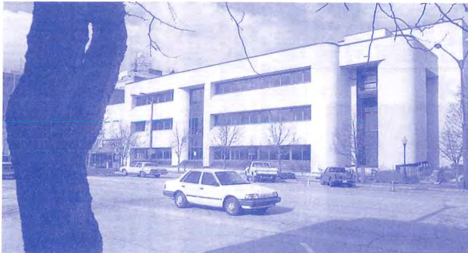
Photo above: At the end of fiscal year 1998, the Retirement System moved to a new location. The newly renovated office building is at 611 South Kansas Avenue in Topeka. The lobby and reception area are conveniently located on the first floor, and are easily accessible to all members. Parking is available outside the front door on Kansas Avenue, as well as in a covered parking garage directly below the office building.
